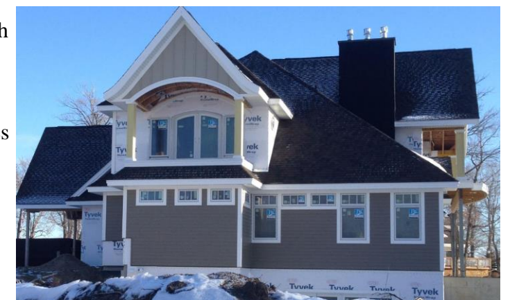
Versatex® Trim Highlights the Curved Roof Lines and Arcs
